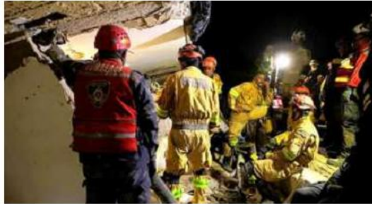
Rescuers at the site of a collapsed building after the June 24 earthquakes in La Guaira, Venezuela, on Thursday. REUTERS
